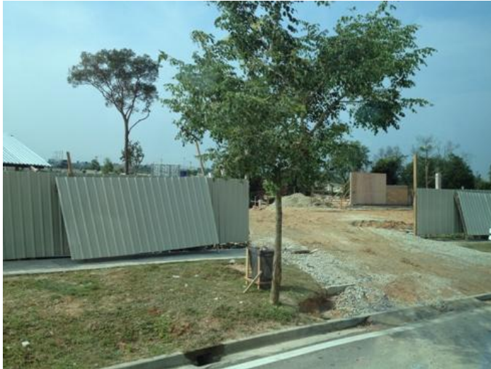
Figure 47: Meridin construction site
