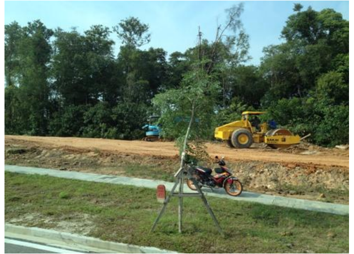
Figure 48: Earthworks being carried out
